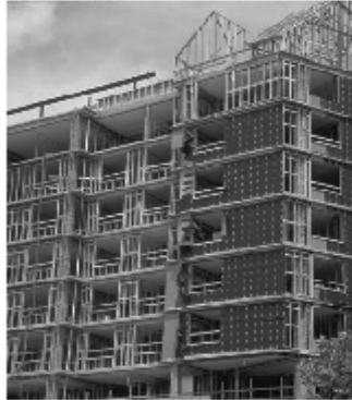
Photo 1 (left): "Harley Davidson" Architecture. The projecting concrete slabs transfer heat across the enclosure. Photo 2 (right): Architectural Statement. Apparently, the projecting slab is visually appealing (who knew?). It catches rain and transfers heat efficiently while wasting floor area (square footage).
