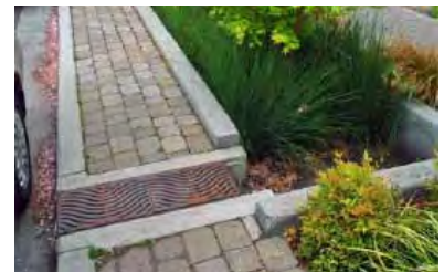
Stormwater filtration beds help filter pollutants from stormwater.
